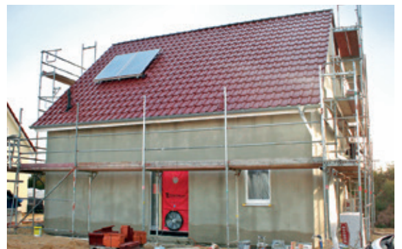
BlowerDoor test of a new single-family home
