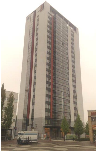
Residential high-rise building: 30.000 m 3
