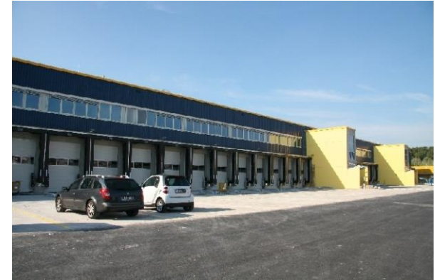
Logistics hall: 40.000 m 3
