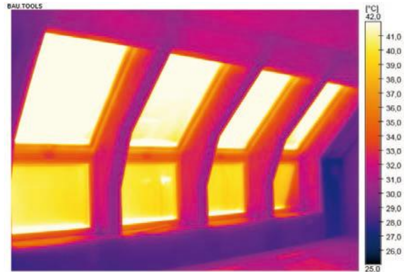
Thermogram of a sunlit window front
